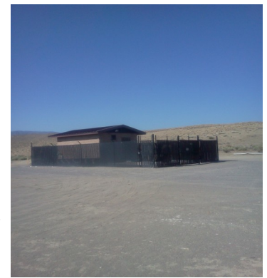
Wadsworth New Municipal Water Well Muni #4
