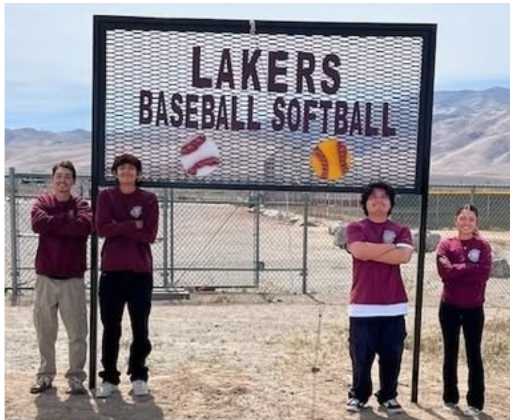
Pyramid Lake JR/SR High School, April 20, 2026: Mr. Estrada's welding students have been hard at work, creating a new build for the baseball and softball field entrance. Great job bringing skill and craftsmanship to improve our campus!
